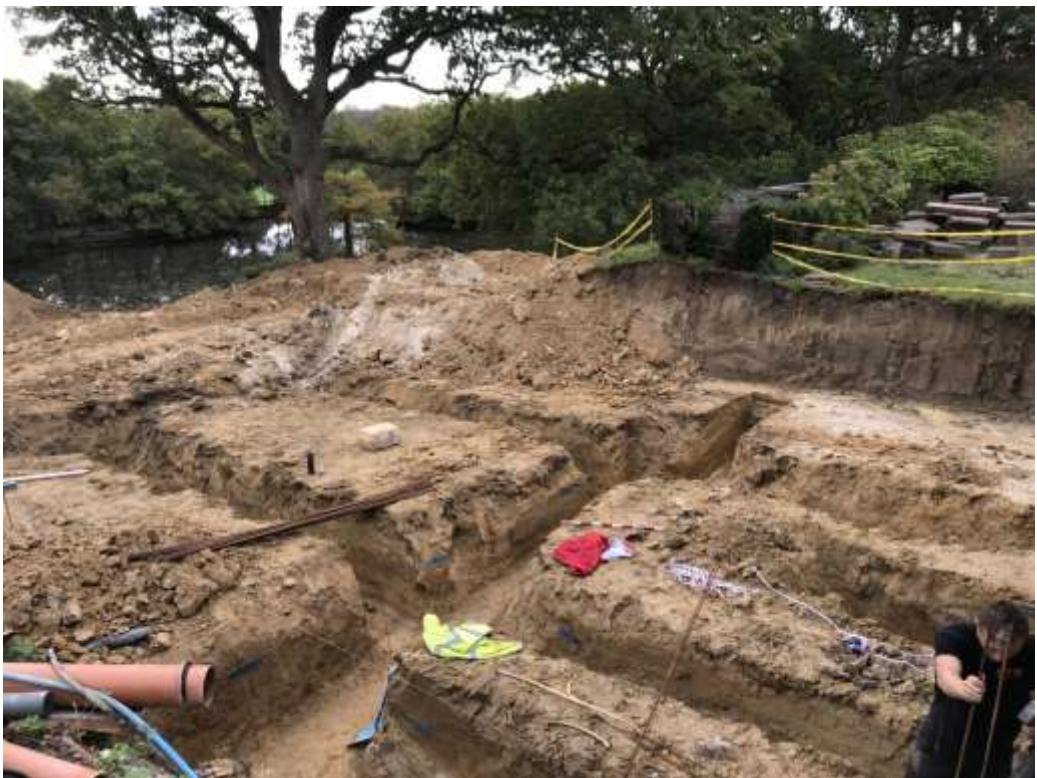
Plate 3. General view of site trenching (looking south)
