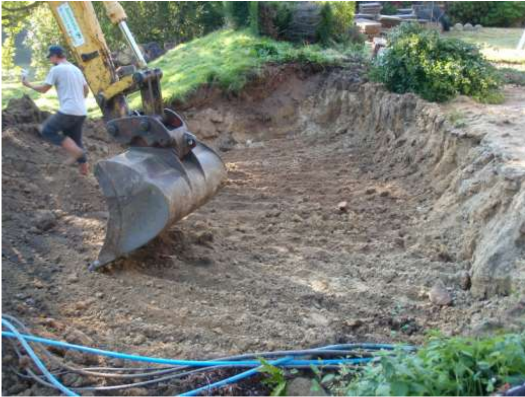
Plate 2. General view of site reduction (looking south)
