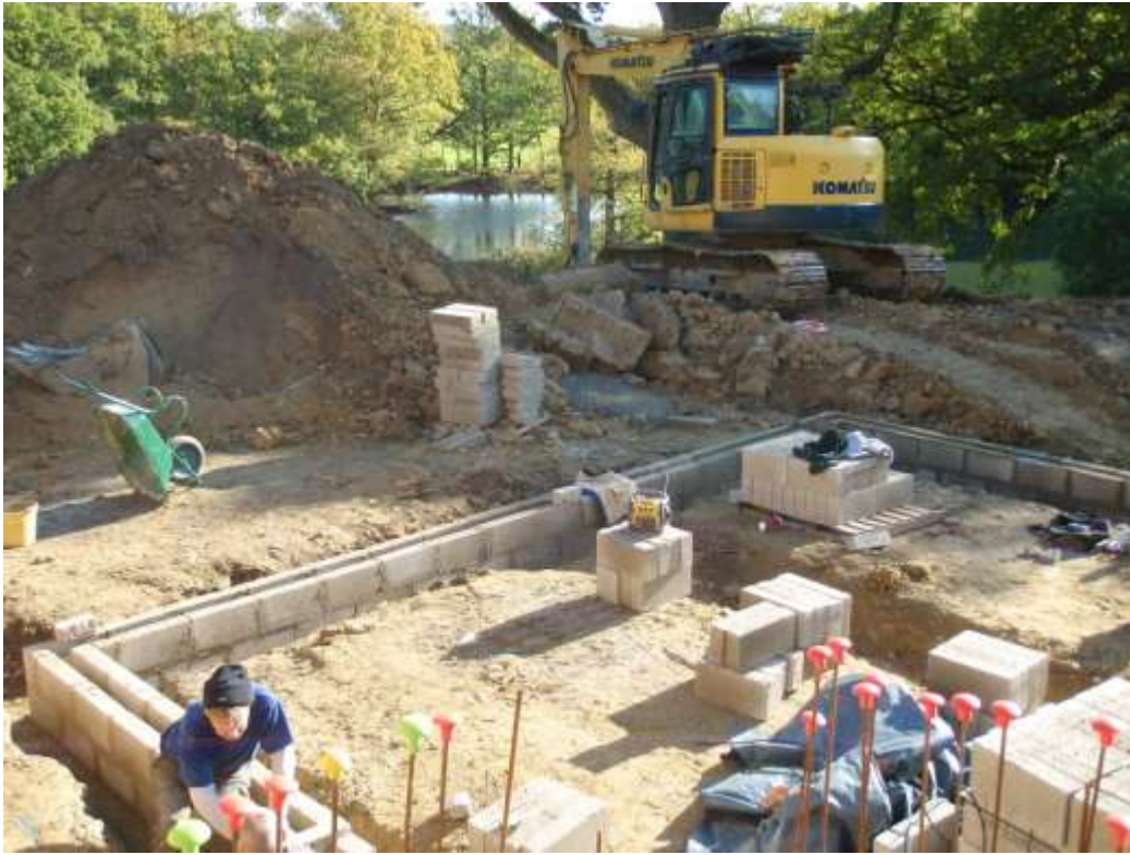
Plate 4. The site showing removing of overburden, trenches completed
